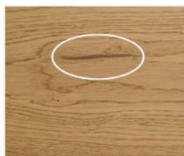
FILLED CRACKS
